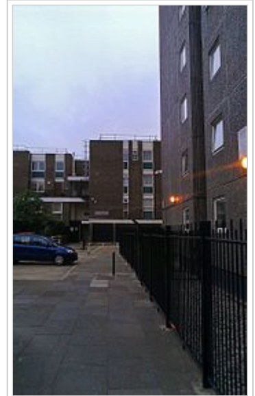
Jeremy Bentham House in Bethnal Green, East London; a modernist apartment block named after the philosopher
